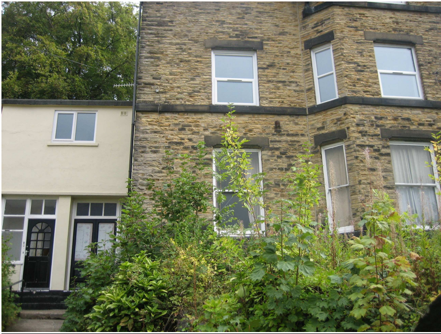
Photographs 2&3 showing the property prior to the installation of the windows
